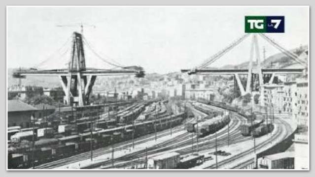
Built in 1963-1967 Great distance 210 m Length 1182 m Concrete prestressed 90 m high Iron cables inside concrete
