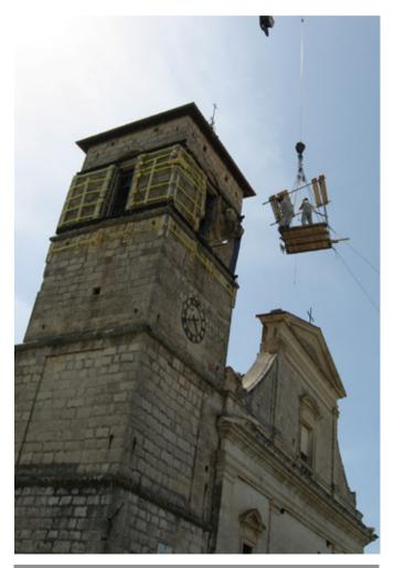
Bell tower of San Felice Martire church in Poggio Picenze (AQ) Piers of the bell tower made of two withes of dressed rectangular stones with debris of smaller size used as fill ( "a sacco" construction). The piers were badly damaged by compression. SAF teams from Tuscany (high angle rope rescue specialists) applied carbon fibres and bi-component fibre-reinforced mortar (fibreglass) to stop the extrusion movement.
