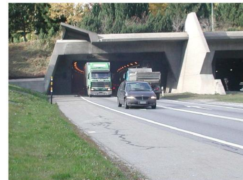
Gotthard Tunnel (CH)
