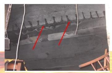
The separation floor with the apartment above was buckled, causing the detachment from the beams
