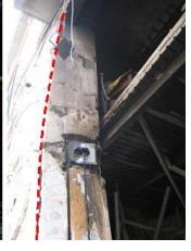
Masonry structures damaged. The outer wall of the building corresponding to the access was visibly damaged to form a convexity towards the outside characterized by various surface fractures of various sizes.
